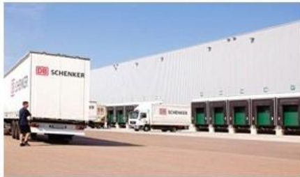
Prologis Park Ausgurg, Munich, Germany
