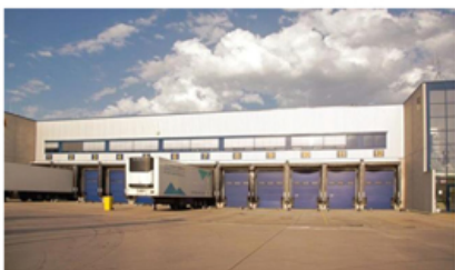
Prologis Park Munich-Neufahrn, Munich, Germany
