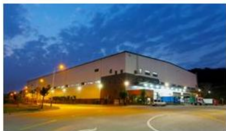
Guangzhou Phase II, Guangzhou, China
