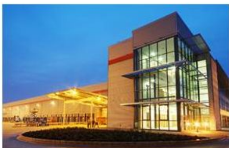
Prologis Swindon, North Hampton, United Kingdom
