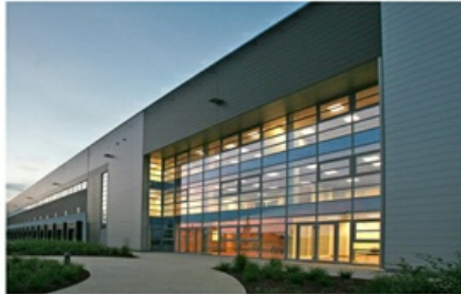
Prologis Park Chanteloup, Cramayel, France
