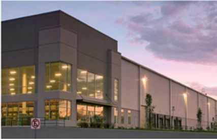
El Salto Distribution Center – Guadalajara, Mexico
