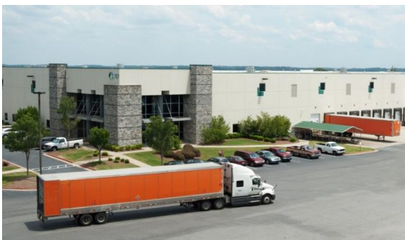
Douglas Hill Park Distribution Center, Atlanta, Georgia, USA
