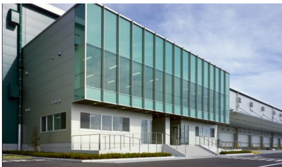
Prologis Park Iwanuma, Miyagi, Japan
