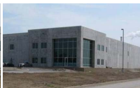
ProLogis Park Rochelle - Chicago (under development March 2011)
