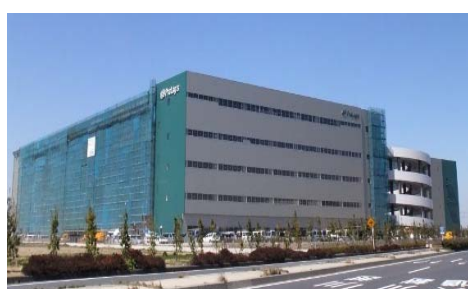
ProLogis Parc Kawajima – Tokyo (under development March 2011)
