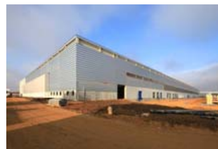
ProLogis Parc Chanteloup – France (under development December 2010)
