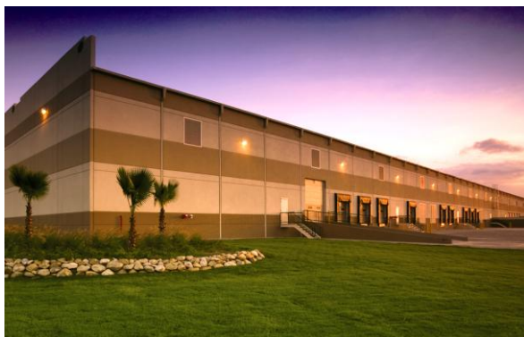
Prologis Park Apodaca, Monterrey, Mexico
